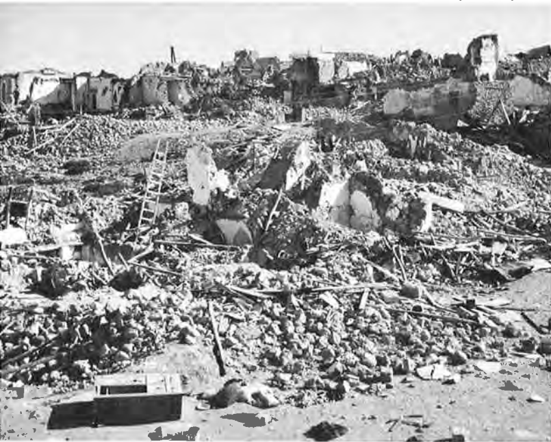
Fig. 15. Collapse of Old Masonry Construction, Yachech District
