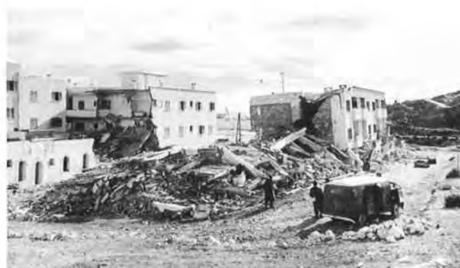
Fig. 22. Collapse of "Modern Appearing" Masonry Construction, Talborjt District
