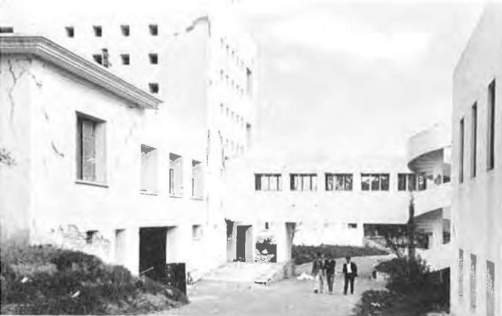
Fig. 26. Lyautey Hospital; Bridge Structure and Spiral Stairway in Good Condition
