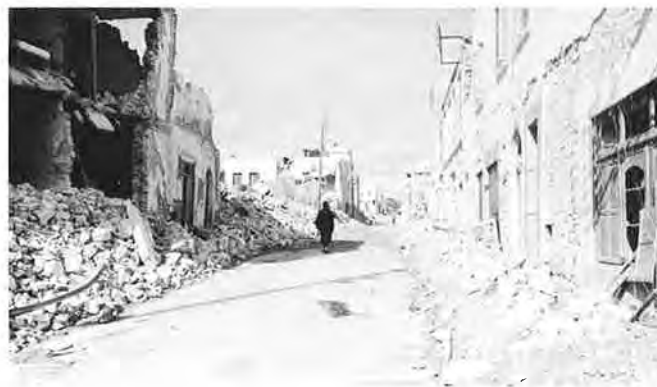
Fig. 21. Scene After Street Has Been Cleared by Bulldozers
