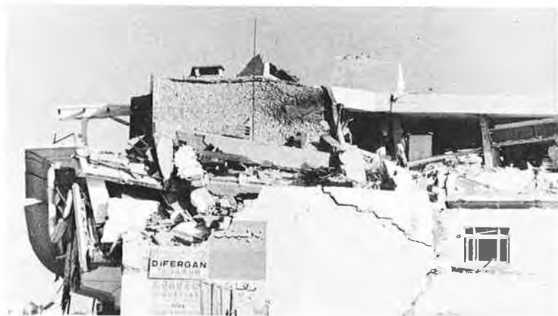
Fig. 51. Sud Building from NE, Overhang of Balcony Is Visible
