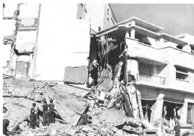
Fig. 31. Collapse of Typical New City Masonry Construction
