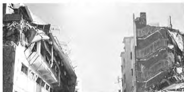
Fig. 32. View of Reinforced Concrete Sud Building on Left, Masonry Structure on Right
