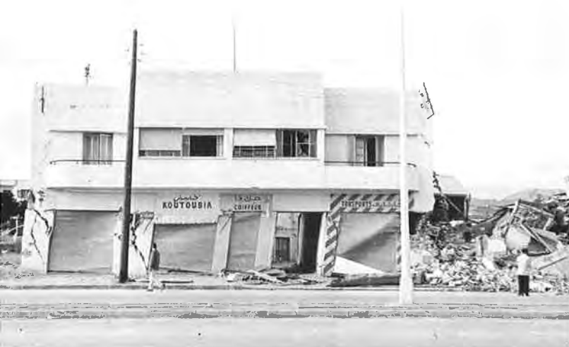
Fig. 35. Racking of Buildings in First Story
