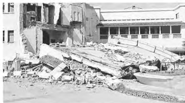
Fig. 34. Damage to Portico of Marhaba Hotel, Typical of Several Examples in Agadir
