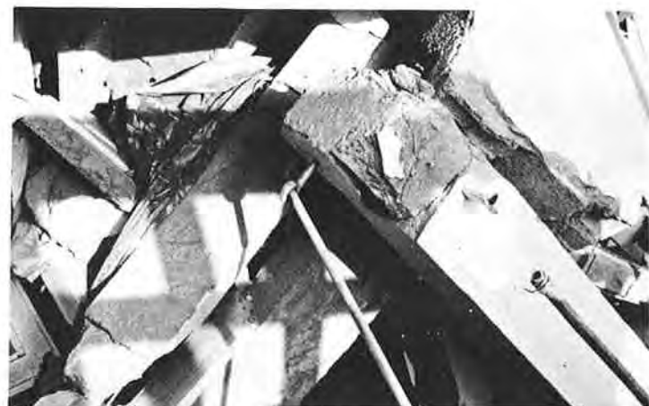
Fig. 48. Saada Hotel Detail, Note Fracture of Beam and Girder
