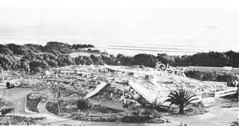
Fig. 45. Saada Hotel from the Northeast, After the Earthquake
