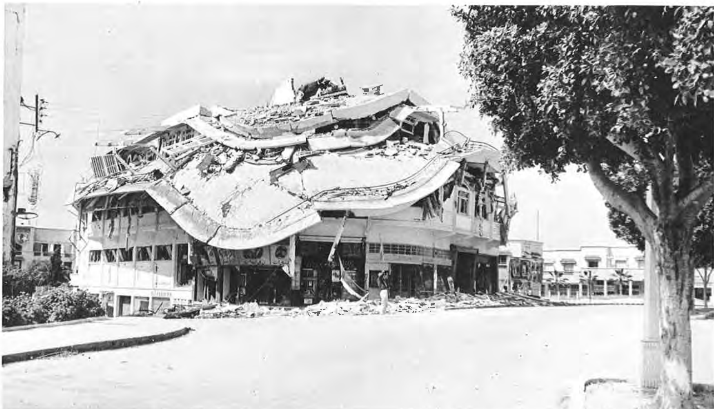
Fig. 49. Sud Building from the Southeast, Third Story Has Collapsed
