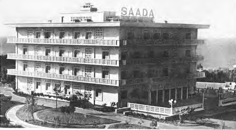
Fig. 44. Saada Hotel from the Northeast, Before Earthquake
