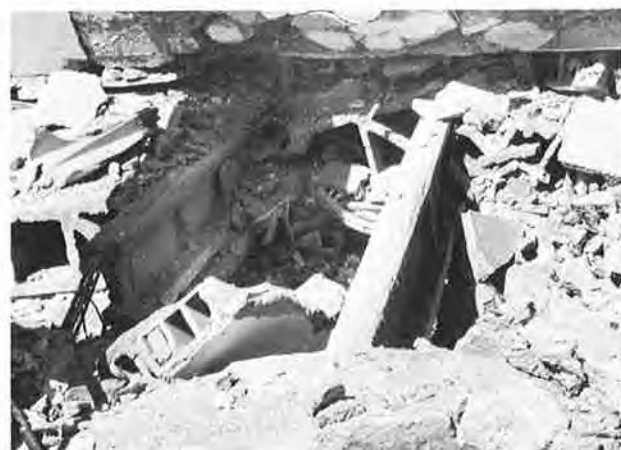
Fig. 43. Precast Floor Beams and Hollow Precast Floor Panels
