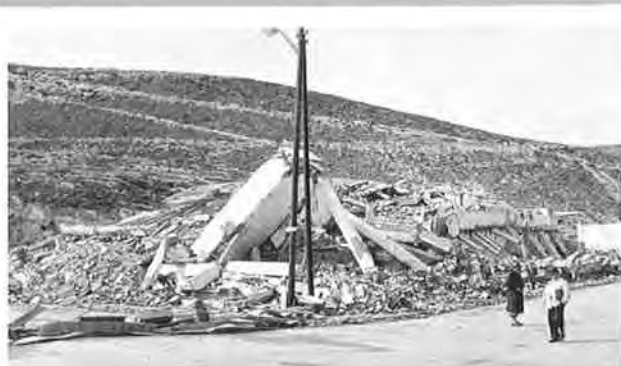
Fig. 40. Immeuble Consulaire from the South, After the Earthquake
