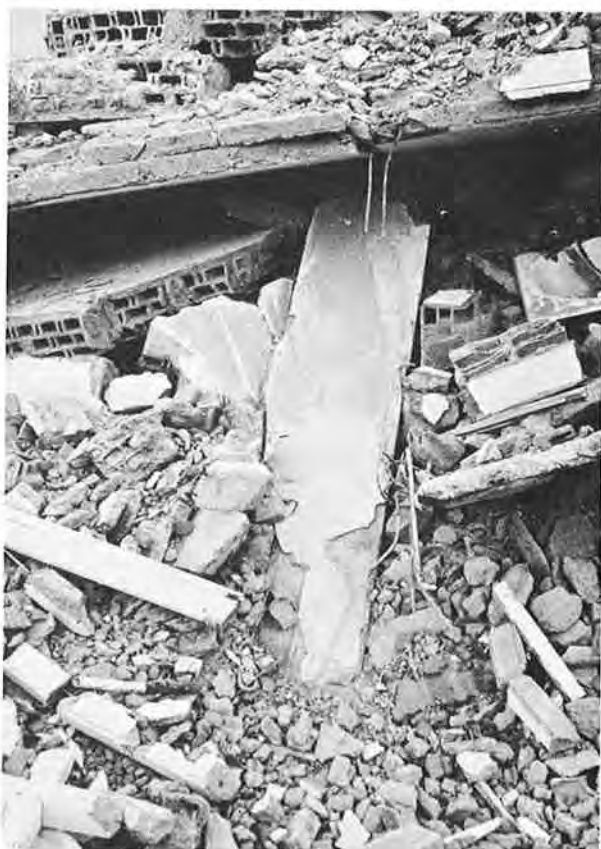
Fig. 46. Hollow Precast Floor Panels of the Saada Hotel
