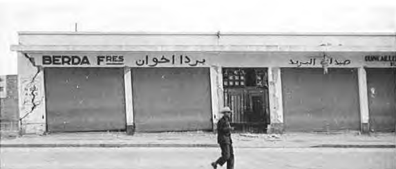
Fig. 36. Note Bracing Effect of Flexible Steel Screens
