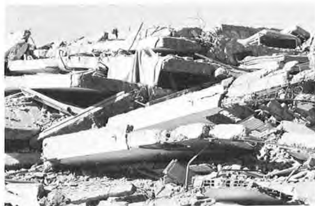
Fig. 41. Immeuble Consulaire, Note the Stack of Successive Floor Slabs
