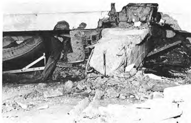
Fig. 47. Saada Hotel Detail, Note Lack of Continuity Between Members
